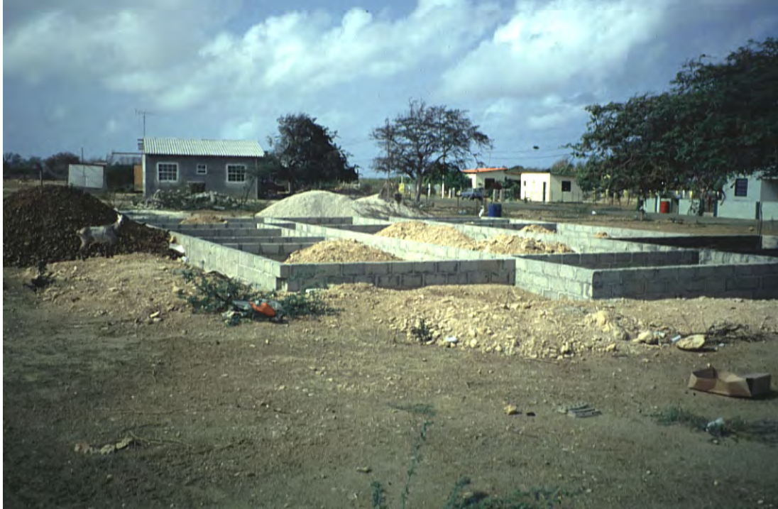
Figure 114: Typical Construction Site
