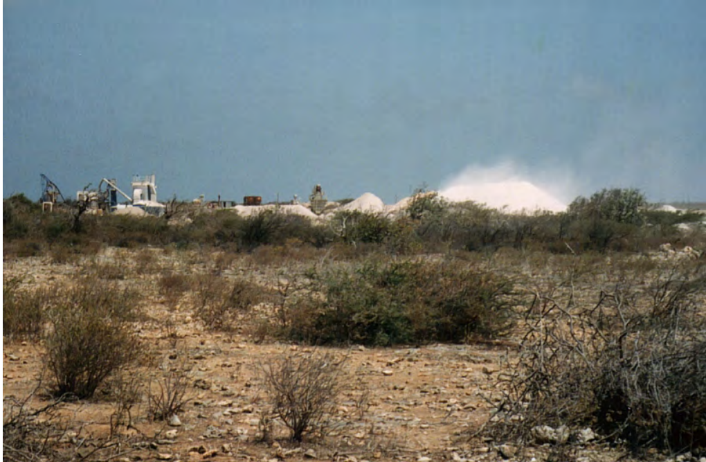
Figure 124: Stone Crushing Plant
