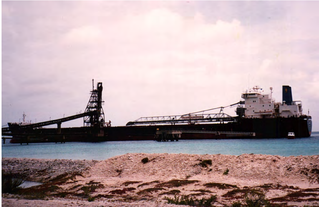
Figure 148: Salt Works Pier The feasibility of the Bonaire salt works is assisted by the steep marine topography that permits near-shore access to ocean-going vessels.
