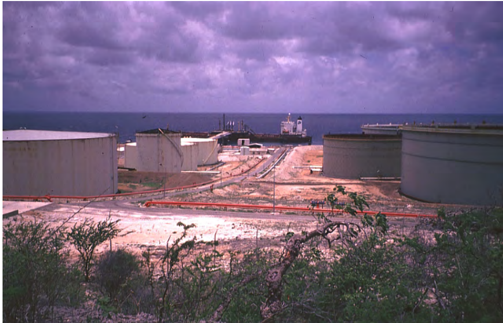
Figure 145: Oil Transshipment Terminal A few of the 23 storage tanks within the terminal. Note the proximity of the ship that is loading (or unloading) crude oil to the tanks. Bonaire's uniquely steep underwater topography permits tankers to moor very close to shore.
