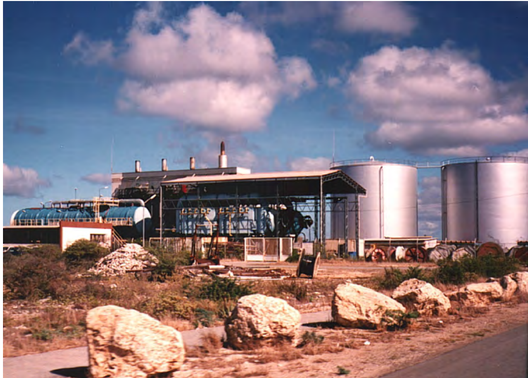
Figure 167: Water and Electric Plant
