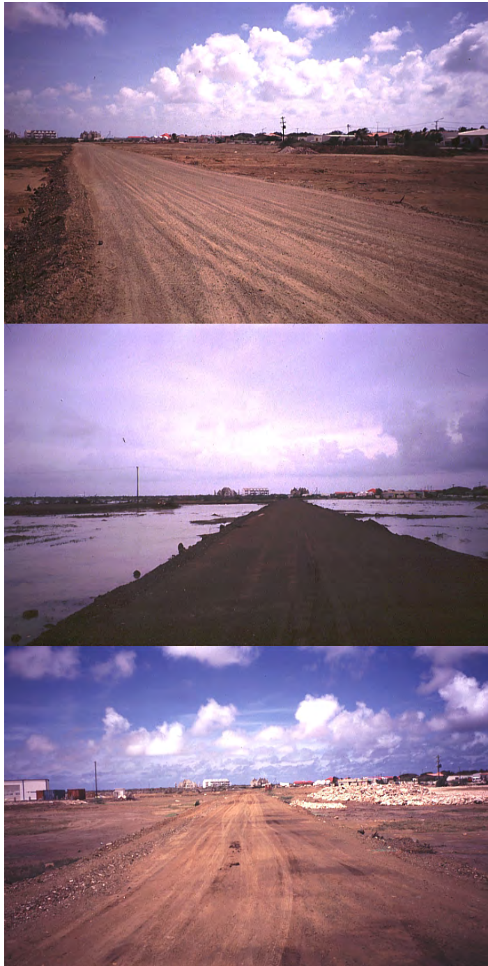
Figure 129: New Road Subbase
