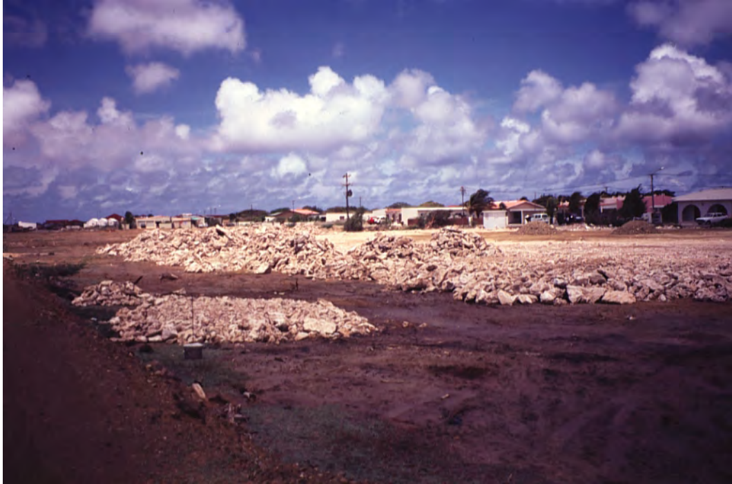
Figure 125: Limestone for Fill
