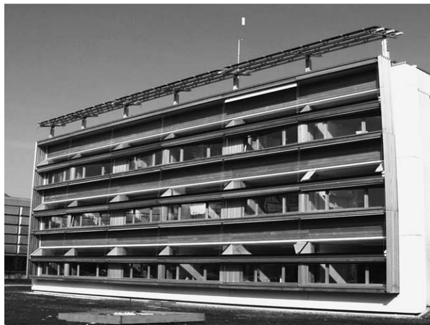
Fig. 1. View of the south facade and photovoltaic installation of the LESO building.
